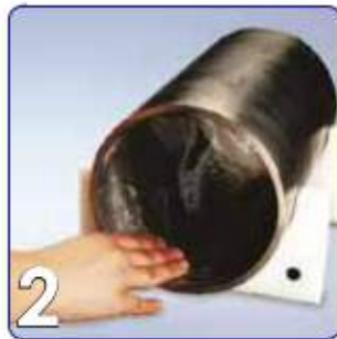
2 Apply LiquiFilm™ Water Soluble Adhesive to inside of pipe
