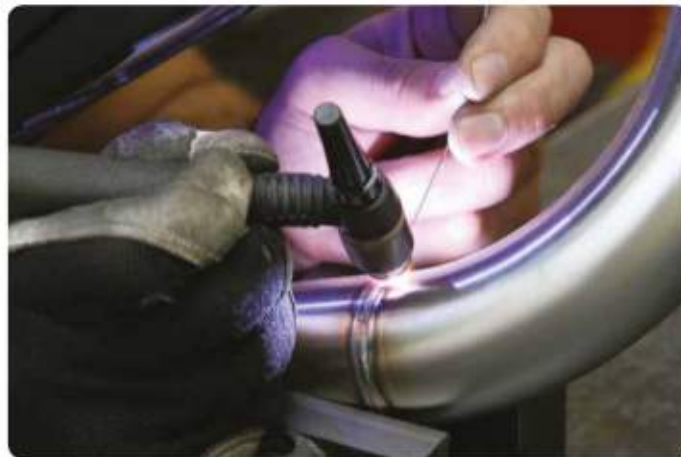
TIG Welding stainless steel elbow
